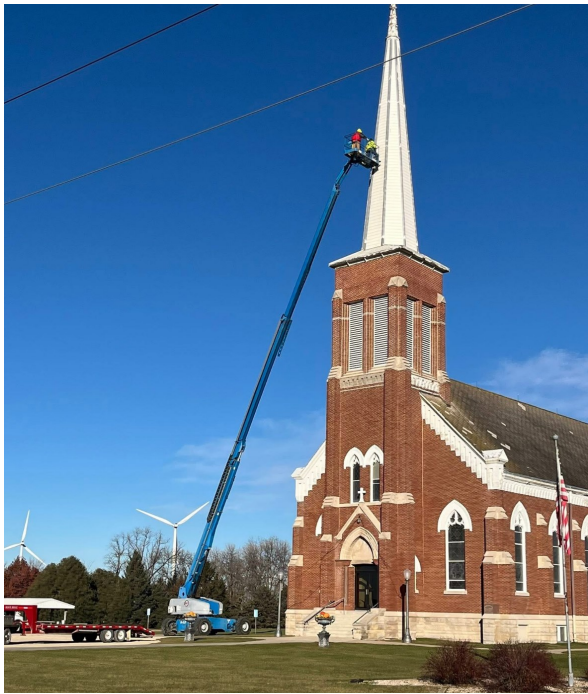
Sacred Heart, Meyer Oratory, steeple repair project.
